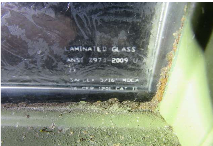
Balance of openings are glazed and all are impact rated - LAMINATED GLASS - MDCA -
