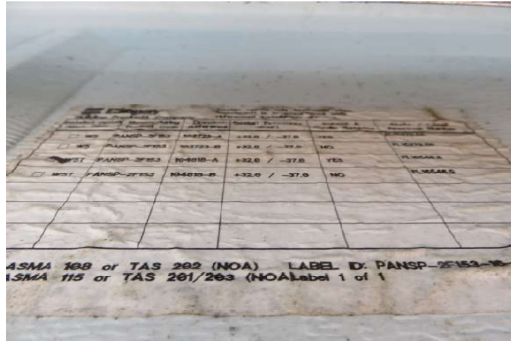
All non-glazed garage doors are impact rated
