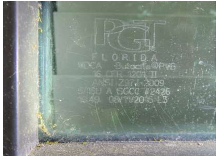
Balance of openings are glazed and all are impact rated - LAMINATED GLASS - MDCA -
